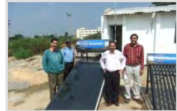
» Installation of solar panels at JAIN University
